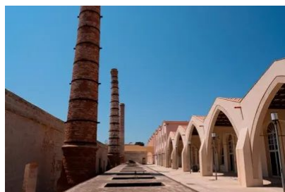
The former Florio tuna factory
