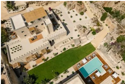
The building inside the excavation, from directly above
