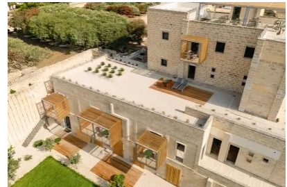
The timber loggias of the houses
